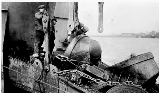
Repair bucket dredger HAM 107 Pernis, around 1950 (source Van Oord).
